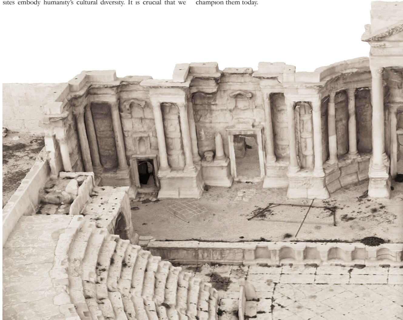
3D model of the Theatre of Palmyra before (left) and after (right) its destruction by the Islamic State.
